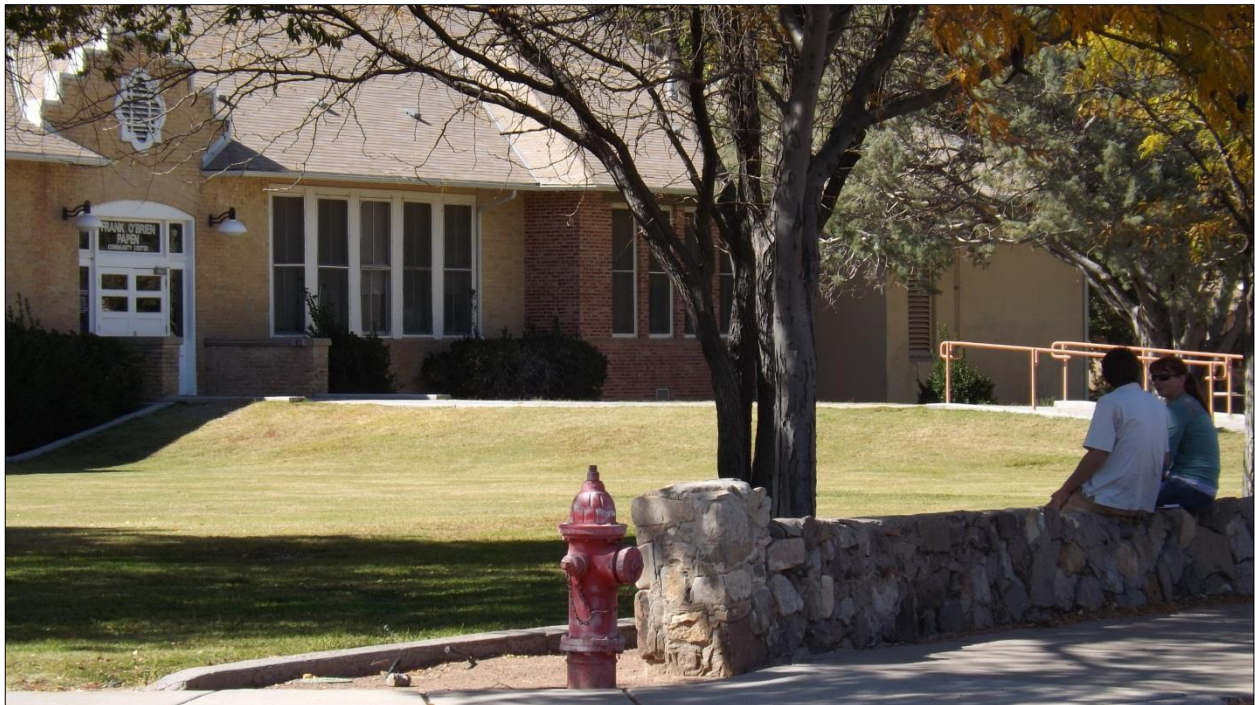
The Frank O. Papan Community Center is an excellent example of adaptive re-use of a historic building. The structure, built in 1900, was used as an elementary school until 1975. The site includes a park, playground and basketball court.
