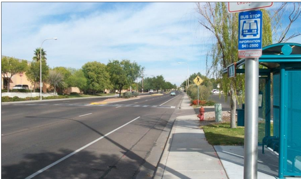
This section of Telshor Boulevard is an example of a Complete Street. It accommodates users of sidewalks, transit and bike lanes.
