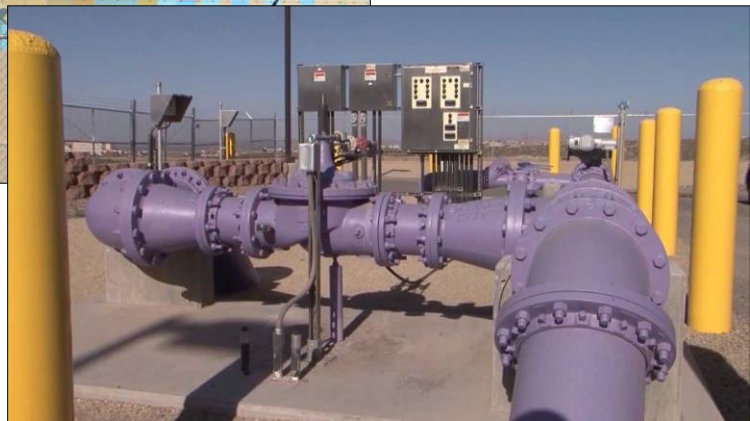
Las Cruces’ East Mesa water reclamation project can provide up to 1,000,000 gallons of water per day through the purple pipe system. The water is half the cost of potable water and is used for landscaping in City parks, private golf courses, and the wetland area behind the Las Cruces Dam.
