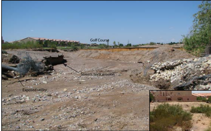
Flooding near the Sonoma Ranch Golf Course inspired a simple and inexpensive naturalistic erosion measure (below) which preserves natural vegetation and blends in with the surrounding terrain. Both photos: CLC Public Works Dept.
