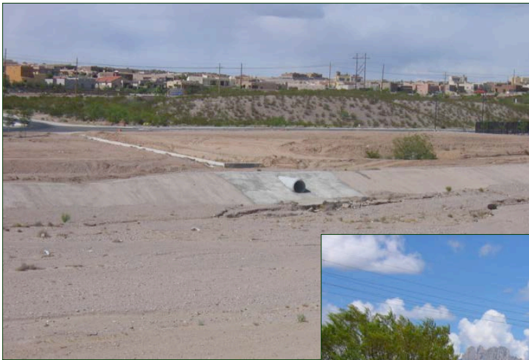
Besides their unsightly appearance, canalized arroyos increase runoff volume and water velocity, thus contributing to flooding and erosion downstream. This is a section of the South Fork of the Las Cruces Arroyo, east of Roadrunner Parkway.
