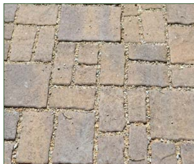
Permeable concrete and pavers allow rain to seep into the ground. Permeable paving can capture and soak in up to 80 to 100 percent of the rain that lands on it and can reduce construction costs for residential and commercial development by reducing the need for drainage features. Photos: www.epa.gov .
