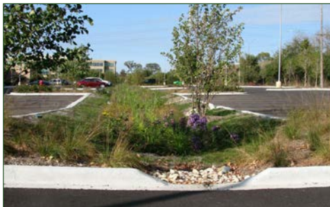
Bioswales are vegetated, mulched or xeriscaped channels that provide treatment and retention as they move stormwater from one place to another. Swales slow, and filter stormwater flows. As linear features, vegetated swales are particularly suitable for draining water from streets and parking lots. Photo: Dave Leonard Tree Specialists, www.dlarborist.com
